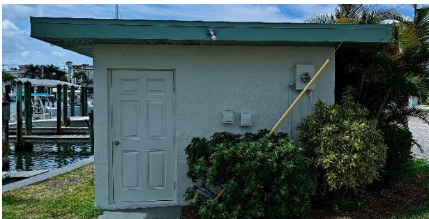
Fig. 16.4 Door to shed storage room (north side)
