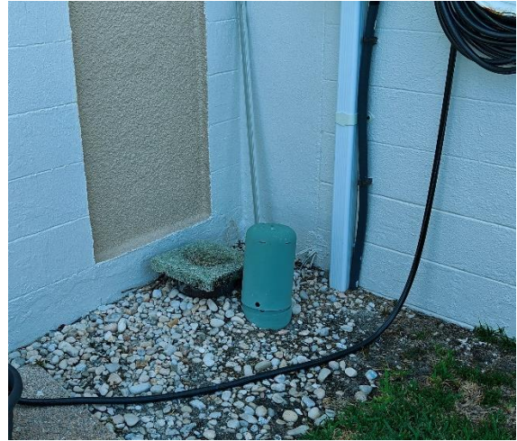
Fig 7.2 Northeast sewer access
