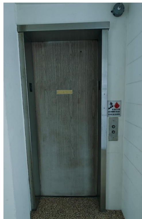
Fig 11.2 Outside elevator door floors 2 - 5
