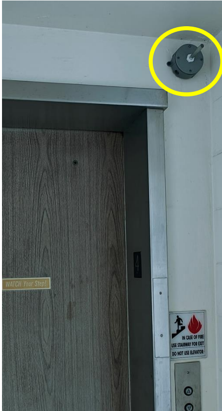
Fig 12.3 Smoke & heat detector
