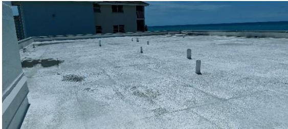
Fig 1.1 Roof looking south
