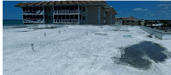
Fig 1.2 Roof looking north
