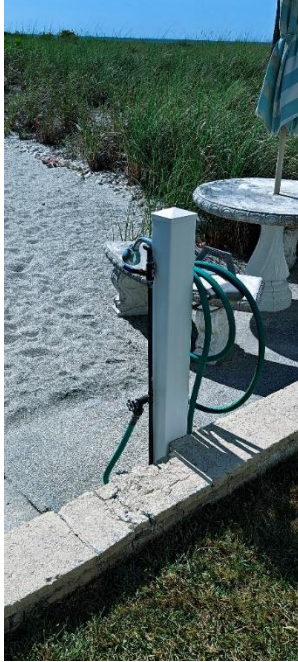
Fig 8.1 Beach water faucet and hose
