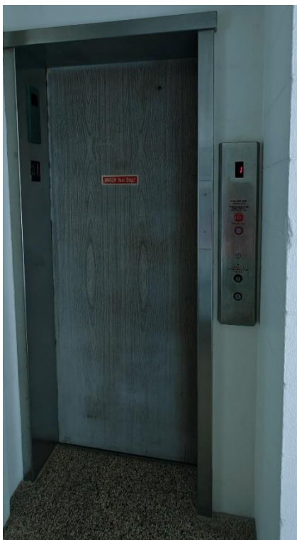
Fig 11.1 Outside elevator door floor 1
