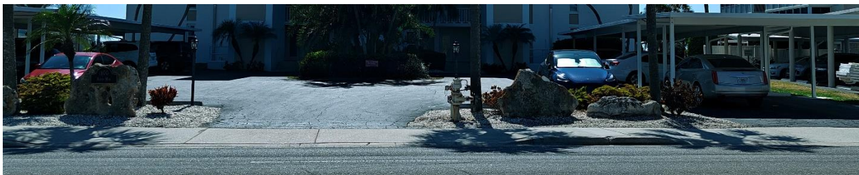
Fig 5.1 Main parking lot entrance with lights
