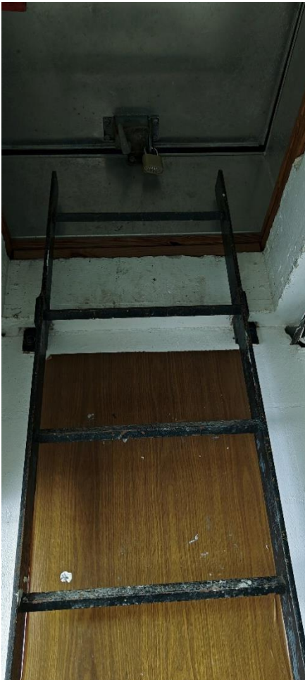
Fig 1.3 Roof hatch door in 5 th floor laundry room - closed
