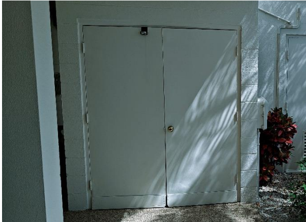
Fig 4.1 First floor storage doors
