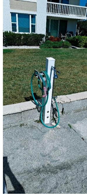
Fig 8.2 Beach water faucet and hose looking toward building
