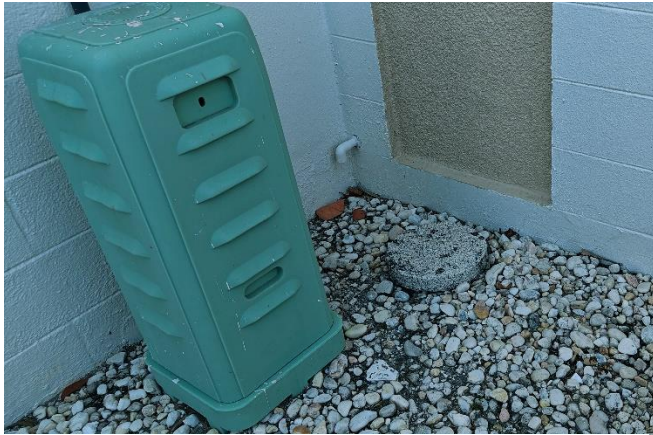
Fig 7.1 Southeast sewer access
